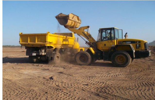
Site preparation including bulk earthworks for Housing Development at Gerehu Heights
